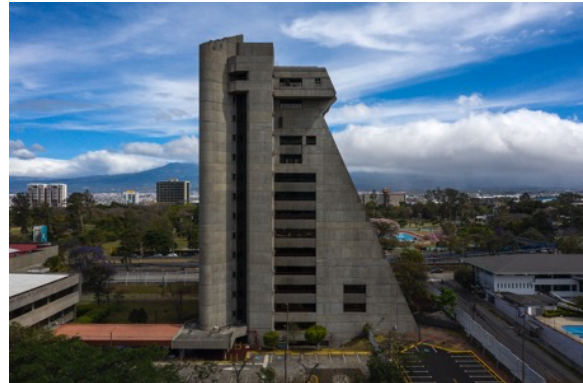
Contraloría General de la República (Office of the Comptroller General of the Republic), San José, Costa Rica, designed by Raúl Goddard, 1980–89. Photograph by Leonardo Finotti, 2021. © Leonardo Finotti
